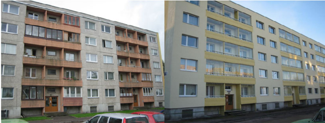
Figure 18. Apartment building at Paldiski road, before and after refurbishment.
