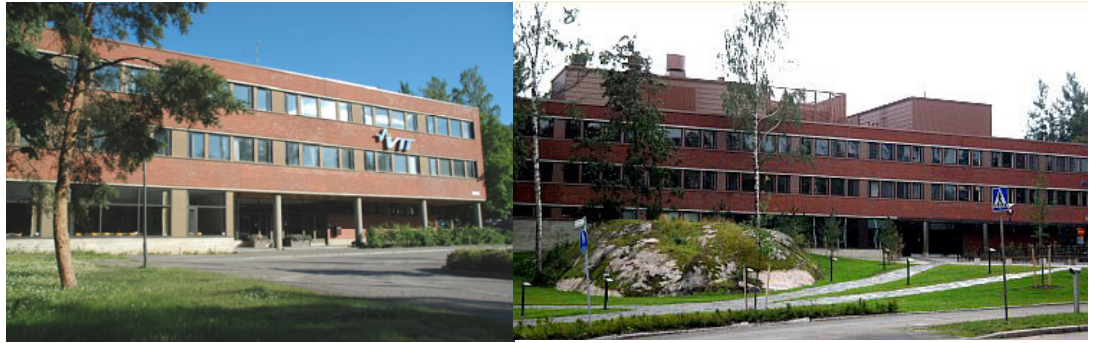
Figure 11. VTT office building before (2005) and after (2007) renovation.
