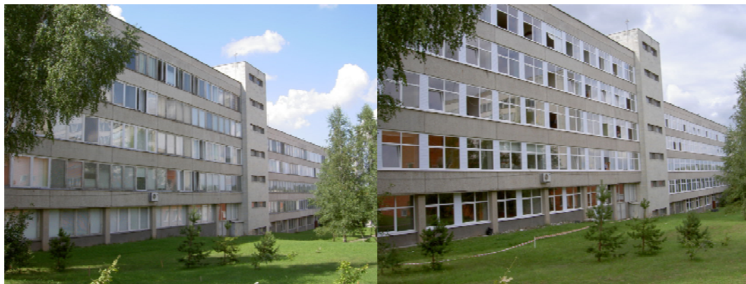
Figure 23. Laboratory Building of VGTU – before and after renovation.
