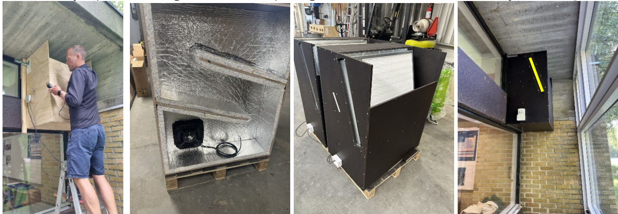
Figure 11. Ventilation box: initial testing, construction, placement of the filter and installation in the DSF.
