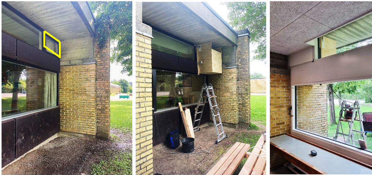
Figure 10. The existing opening, highlighted in yellow and the ventilation box mounted to the existing façade (exterior and interior view).
