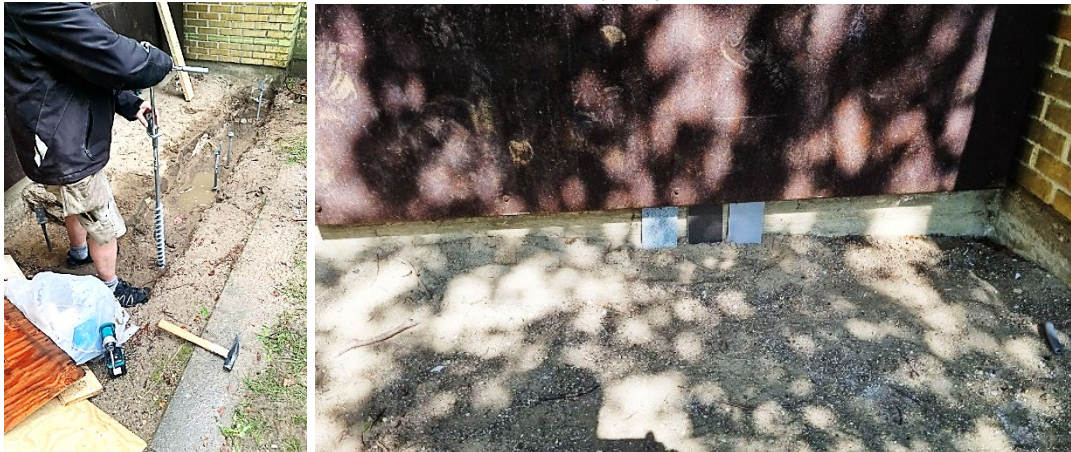
Figure 15. Placement of screw foundation and selection of color palette.
