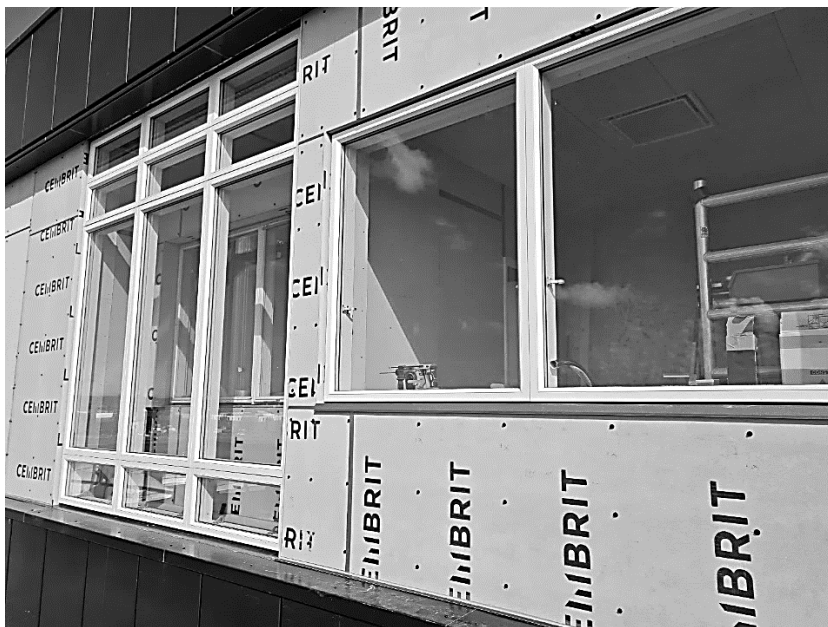
Figure 7. The photo illustrates the facades of two rooms at the AAU laboratory. The room on the left features the I-DIFFER solution, while the room on the right represents traditionally renovated facade.
