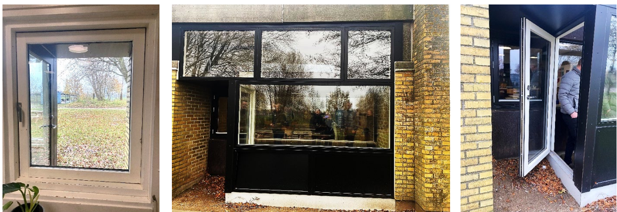
Figure 13. Preserved fire escape opening (inside and outside view). Access to DSF for maintenance.
