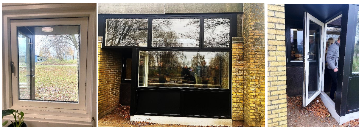
Figure 11. Preserved fire escape opening (inside and outside view). Access to DSF for maintenance.
