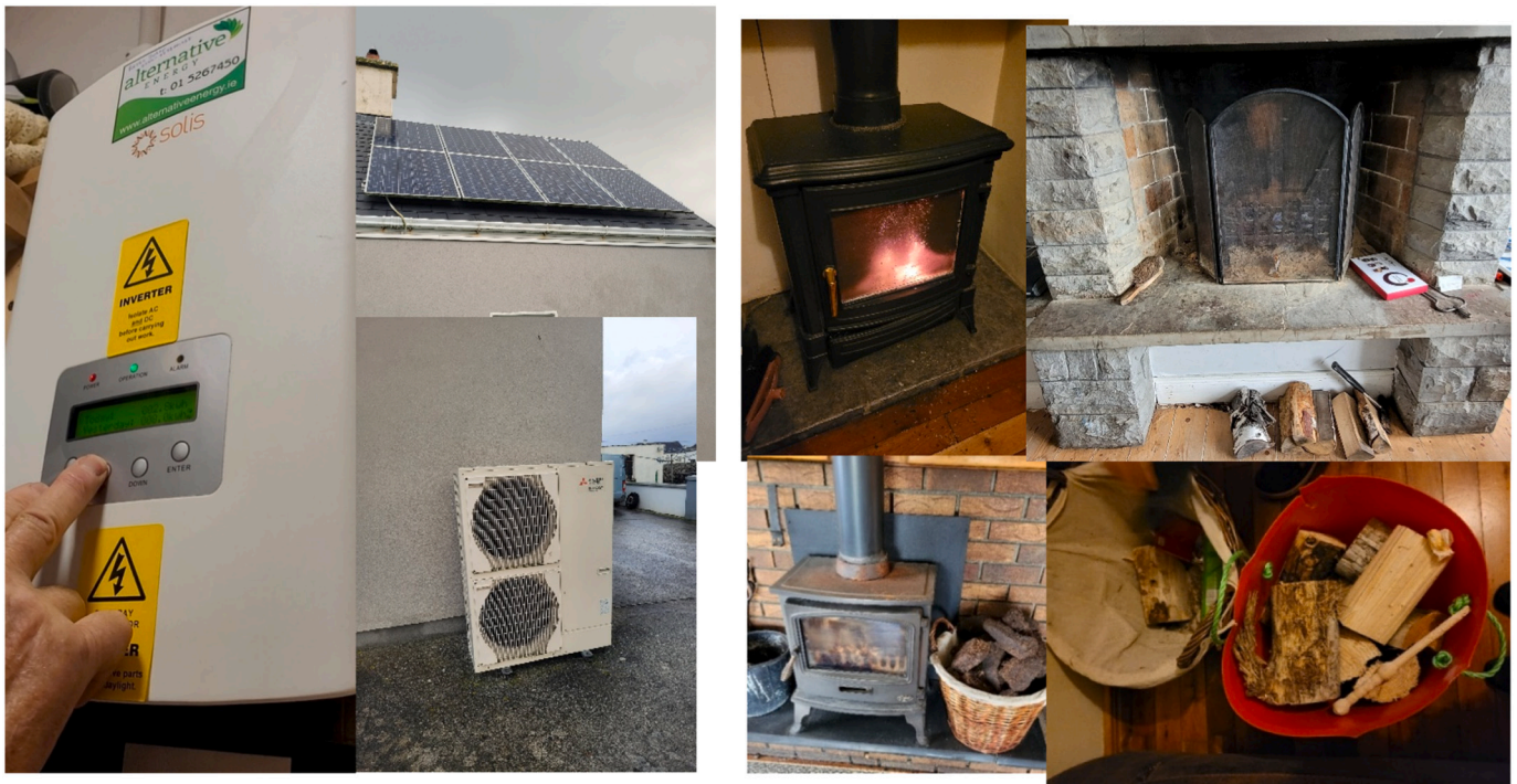
Fig. 3. On the left, examples of solar inverter, solar PVs and heat pump; on the right, examples of different heating sources (stove and fireplace, turf and wood) from households on Inis Mór and Inis Oírr.
