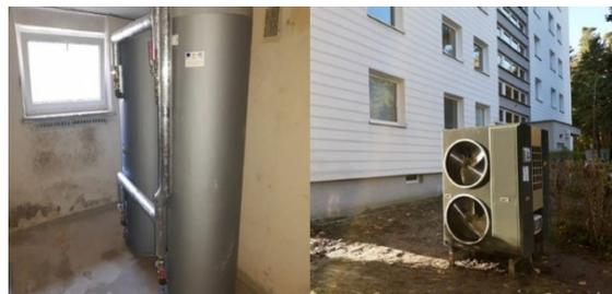
**Figure 7.** DHW (Domestic Hot Water) tanks and GSJ 46EVI HP in the Polish demonstration site
