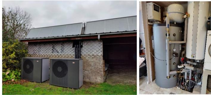
**Figure 4.** Installed HPs and thermal storage on the Danish demo site
