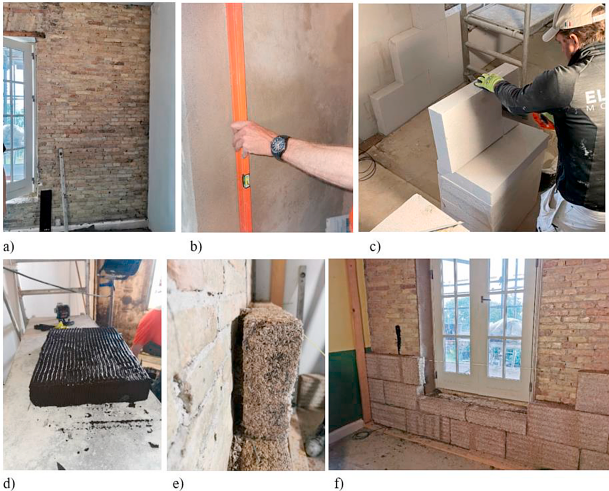
Fig. 7. Photos from the installation of the studied insulation systems. a) Existing wall was cleaned for all old plaster, wall paper and dust, b) New mortar plaster was used to make an even underlay for the insulation (except for system HL), c) Cutting and installation of system AAC, d) Bitumen based glue on system GF was difficult to work with, e) System HL was installed without new mortar plaster as the uneven void between boards and the wall was filled in with HL as a wet granulate, f) System HL under construction also showing the partition wall.
