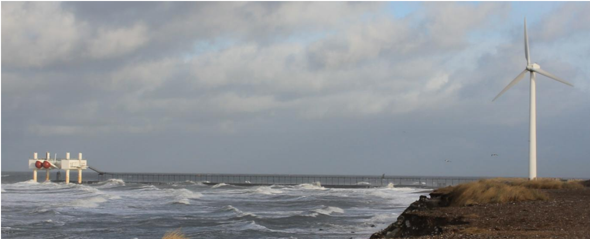
Figure 100. Wavestar (on storm protection mode) and Folkecenter wind turbine at Hanstholm, Denmark.
