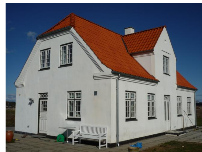
Older detached houses: In the winter 1994-95, measurements of the radon concentration was made in Danish detached residential buildings, built with a slab on ground with a high radon concentration. They showed that 7.7% of these dwellings had a radon concentration in the indoor air above 200 \text{ Bq/m}^3 , and 15.6% had a concentration above 100 \text{ Bq/m}^3 [6]. Measurements were made in 270 detached residential buildings constructed before 1995.
