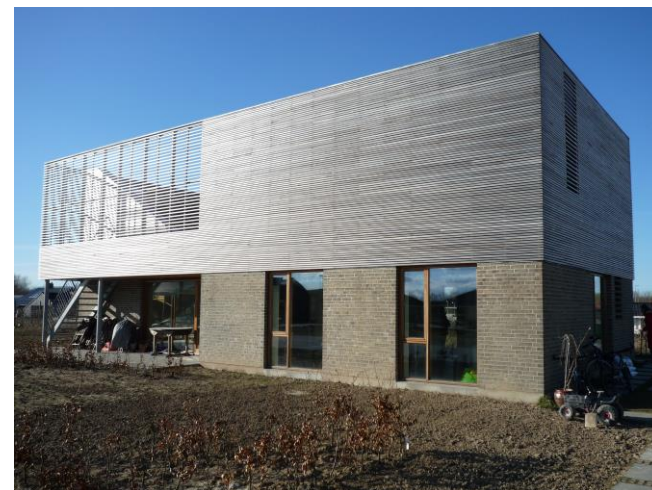
New detached houses: In 2007, measurements of radon concentration were made in new Danish detached residential buildings, constructed with a slab on ground with a high radon concentration. They showed that 1% of these dwellings had a radon concentration in the indoor air above 200 \text{ Bq/m}^3 , and 7% had a concentration above 100 \text{ Bq/m}^3 [5]. Measurements were made in 200 detached residential buildings constructed between 2005 and 2007.
